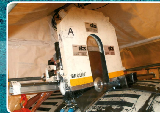
Cuts done by mobile Cold Cutting Saw
